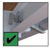
Ensure wind-locks are engaged before moving onto the deck levels.
